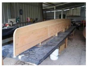
The floats are removed from the frame and taped inside. The floats were levelled and the bulkheads trimmed to fit. All the bulkheads are taped in the floats. A stringer was added in the centre to help the deck hold its shape
